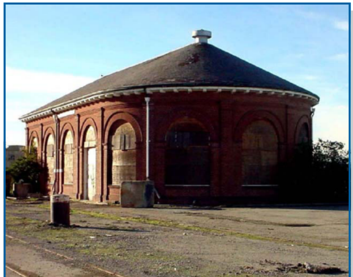
Building 140, Dry Dock 3 Pump Station, Historical Structure
